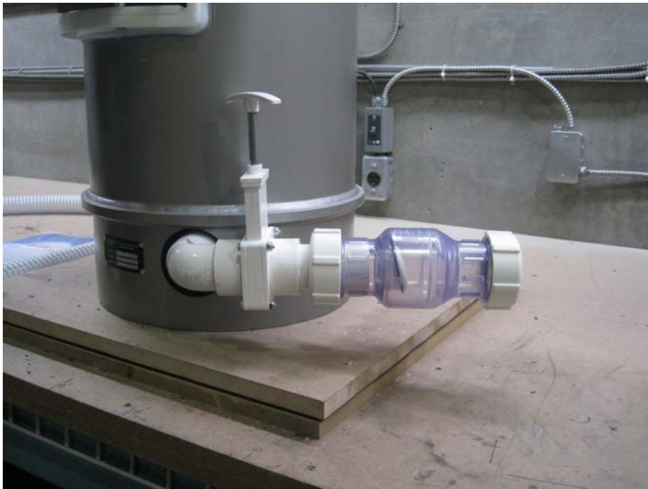
Gravity drain fittings to be connect to floor drain
